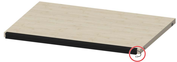
Figure 2. Laying the Floor Panel
