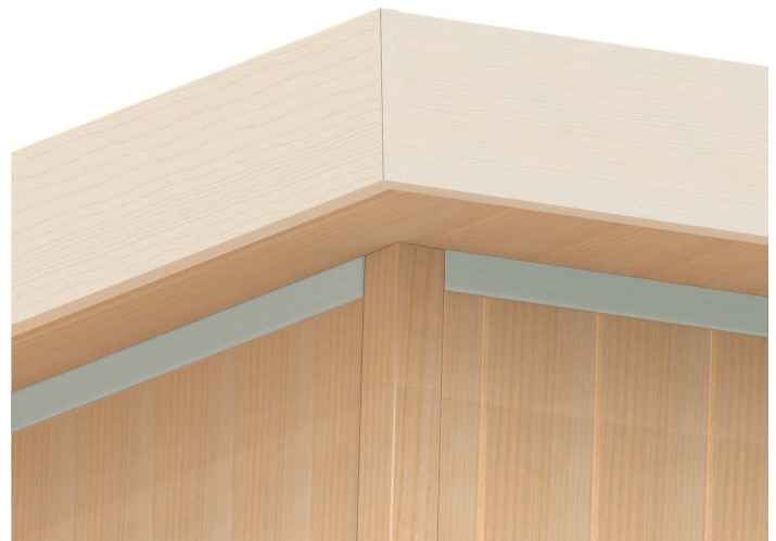
Figure 25. Installing Exterior Cove Trim
