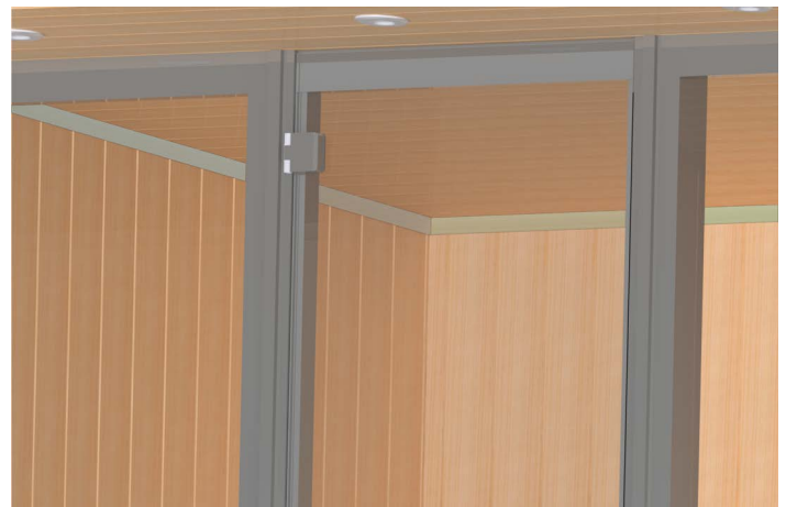
Figure 26. Installing Interior Cove Trim
